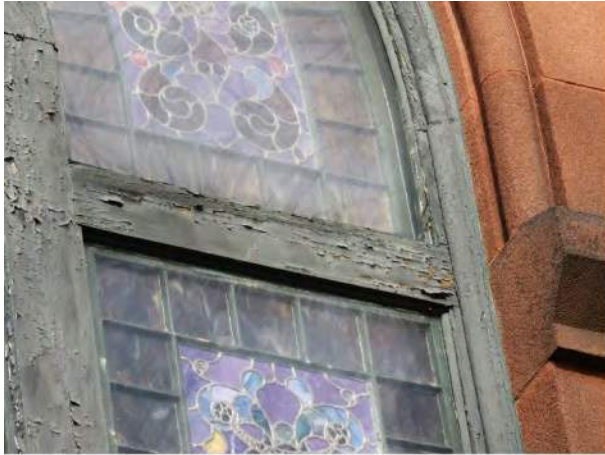
More examples of peeling paint on the frame.
