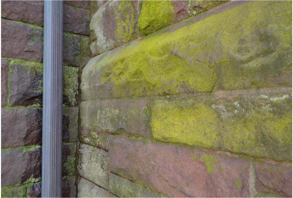
Figure 18 - Biological growth should be removed from the building using the gentlest possible means.
