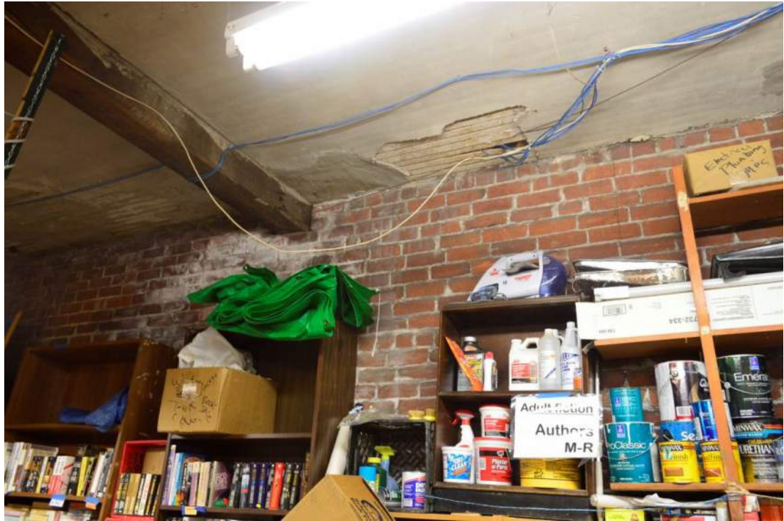
Figure 28 - The failing lath and plaster ceiling should be removed and a fire rated ceiling finish installed.
