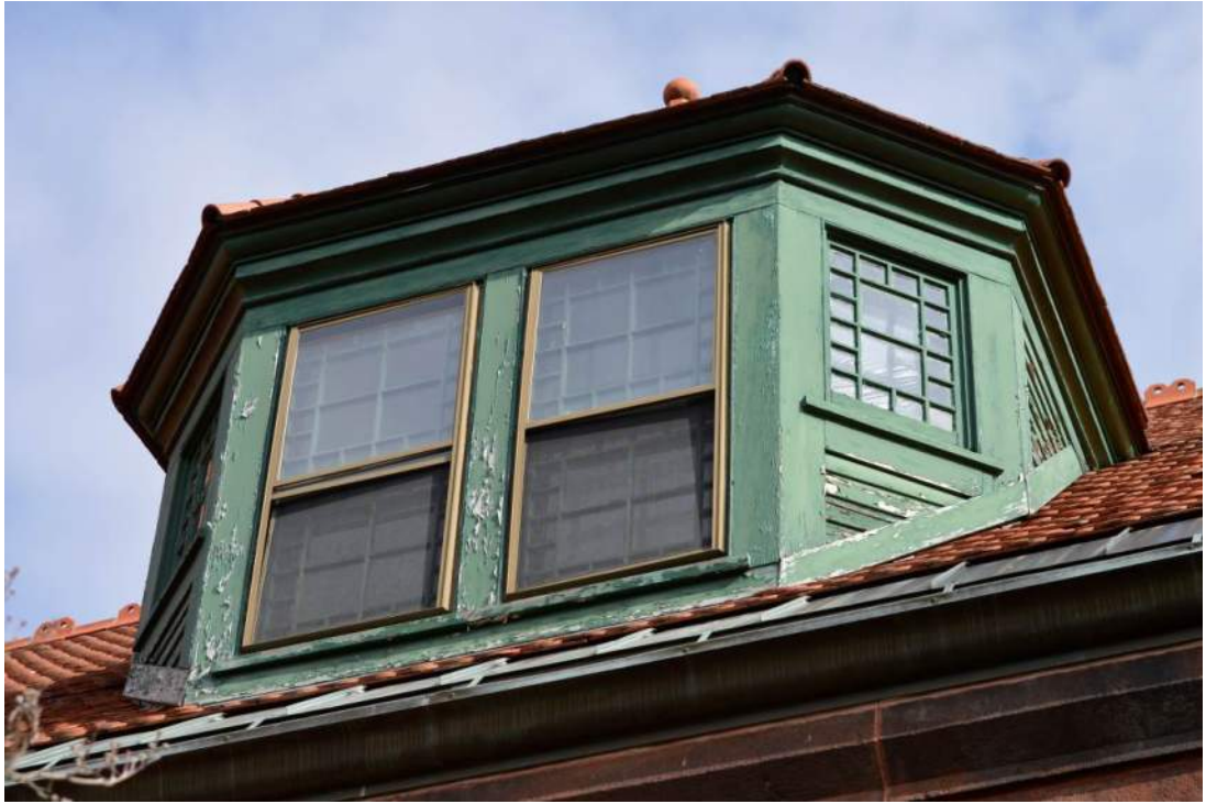
Figure 23 - Wood gable elements require repair and repainting.
