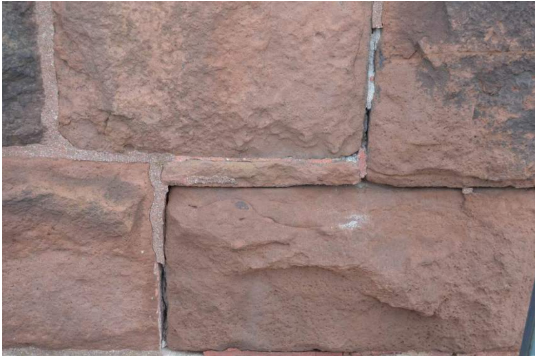
Figure 16 - Past repointing is visible as are stress cracks due to settlement. Areas requiring repointing are limited but occur throughout the facade.
