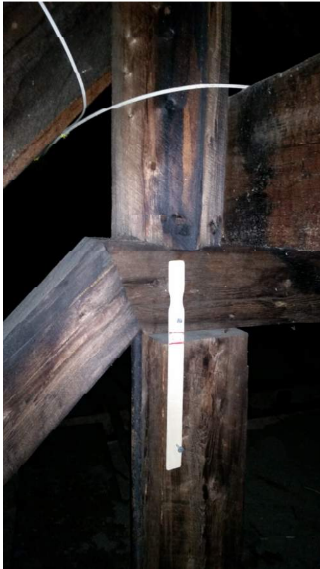
Figure 31 - A telltale has been installed on the King Post truss in the attic to measure movement of the joint.
