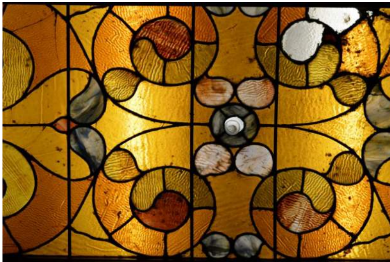
Figure 30 - The central lay lite is slightly damaged. Protective glazing should be installed on the underside.
