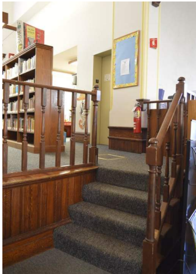
Figure 26 - Stairs to the Children's Reading Area should be rebuilt to have a code compliant rise and run.
