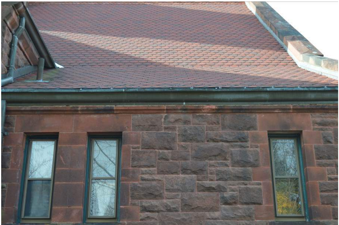
Figure 14 - The asphalt shingle roof on the rear of the building is a substitute for the original clay tile roof. This roof is 20 years old and will be in need of replacement in the next 10 years.
