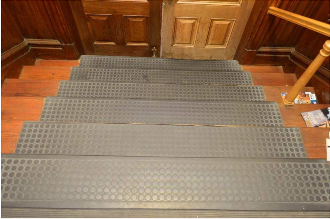
Figure 25 - There is no landing at the base of the front entrance stairs leading to a hazardous condition.
