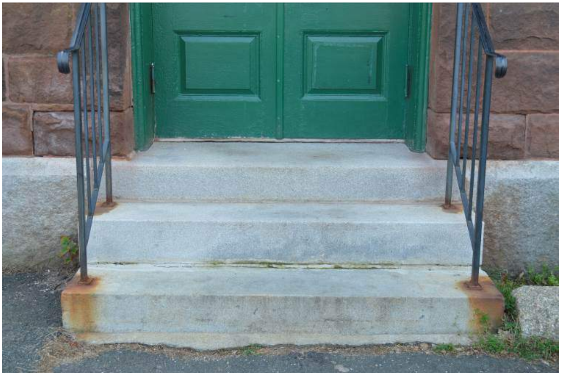
Figure 20 - Rust should be removed from wrought iron railings to prevent spalling of the stone.
