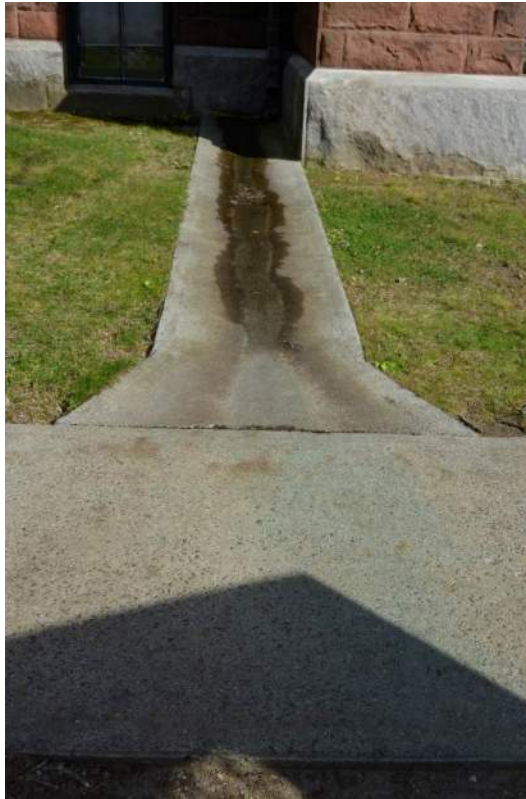
Figure 12 - Surface drainage should be channeled underground to eliminate runoff across walking surfaces.
