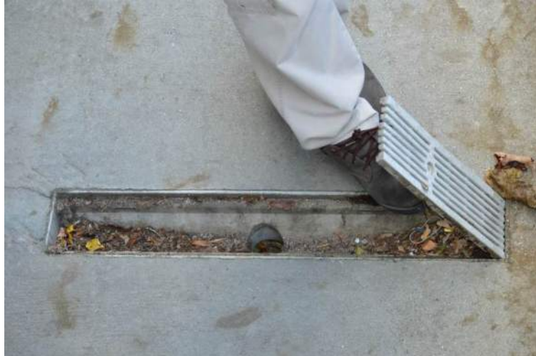
Figure 10 - A trench drain at the base of the entrance ramp requires vigilant cleaning to function properly.
