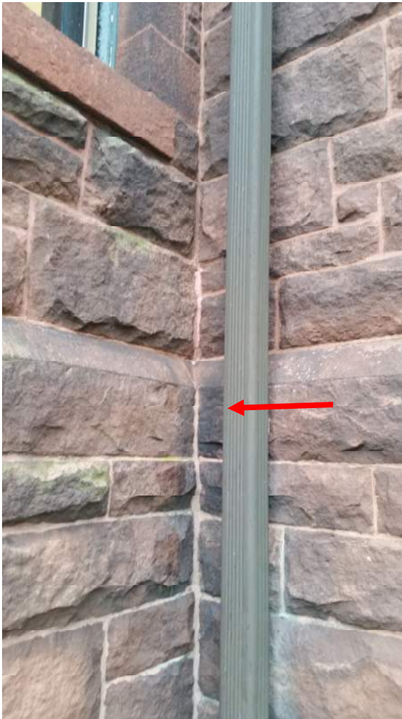
Photo 4: South Interior Corner Near Front Entrance Note past joint repairs on interior corner (sign of past expansion crack repairs)
