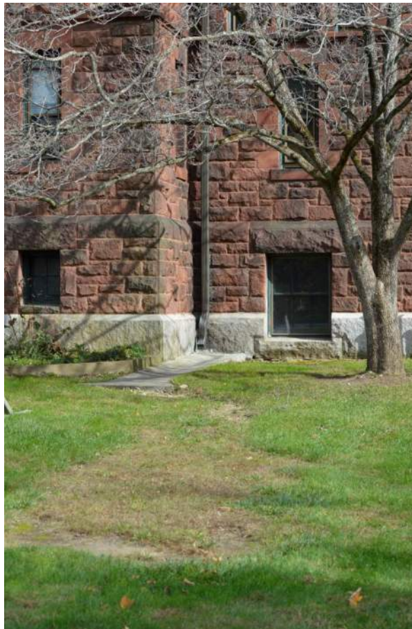
Figure 9 - Roof drainage systems empty across the lawn and the north entrance walk.
