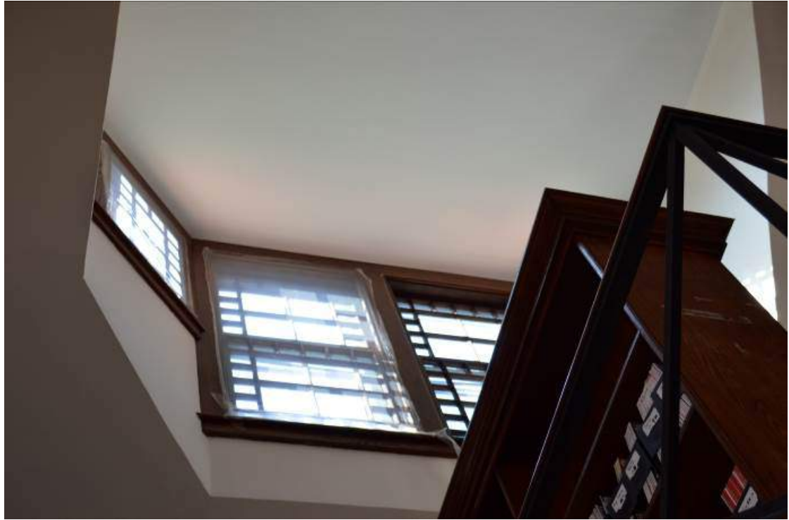
Figure 22 - Interior storm window treatments should be avoided as condensation will occur on the coldest layer, in this case the wood window itself, causing damage to the wood.
