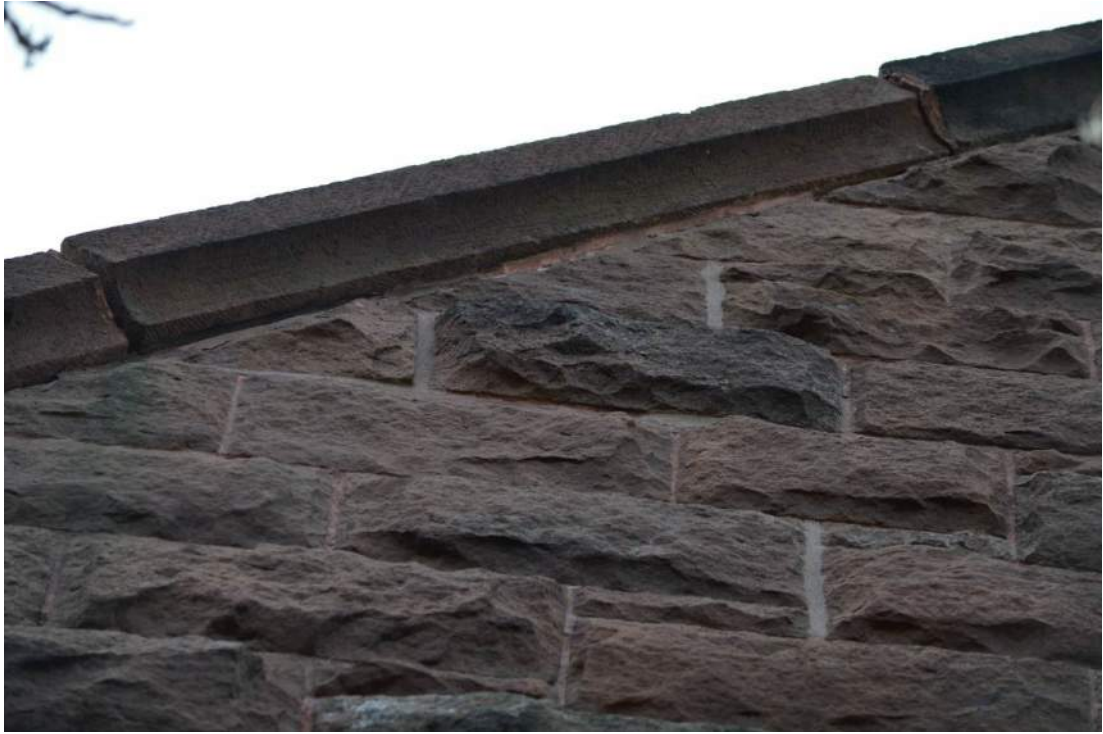
Figure 17 - Displaced coping stones on the gable ends should be reset and re-mortared.
