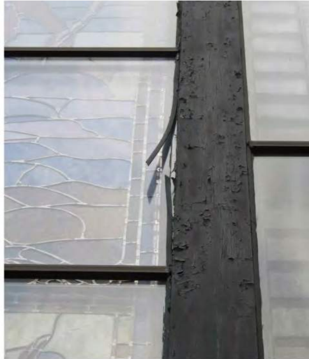
The protective glazing is held in on the side with quarter-round moldings. These are also peeling, as well as splitting and warping.
