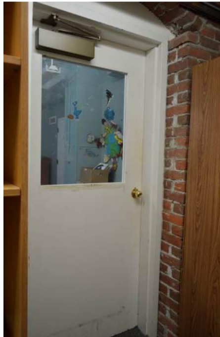
Figure 24 - Door hardware along accessible routes should be code compliant for universal access. In this case a level handle lockset is appropriate.
