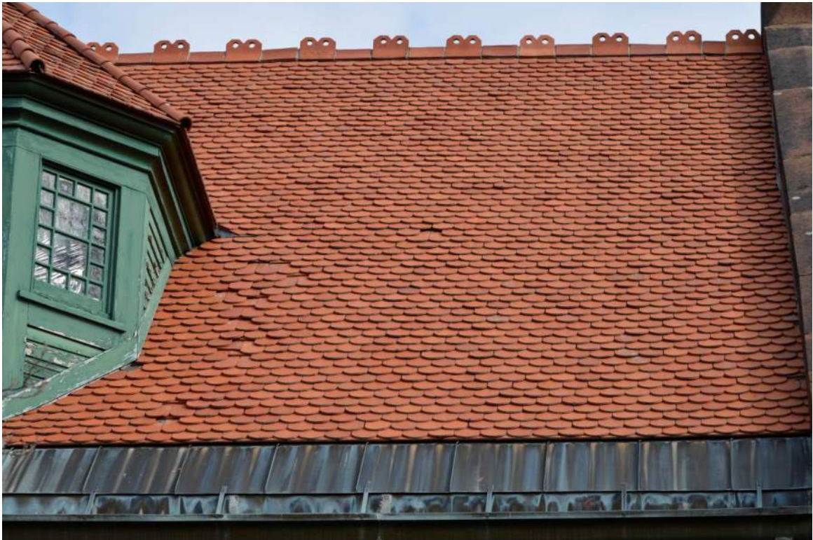
Figure 13 - Clay tile roof shingles are decorative and also fragile.
