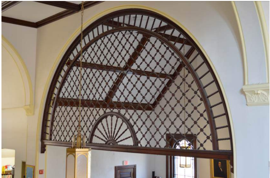
Figure 27 - The decorative screen shows signs of bowing but is not in danger of failure.
