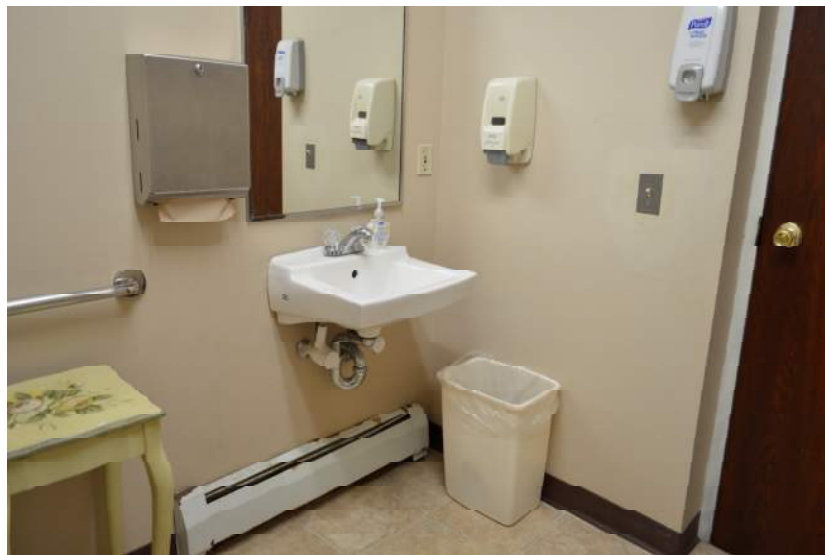
Figure 32 - The heating unit should be replaced, under sink piping should be insulated and dispensers should be mounted at code compliant heights.
