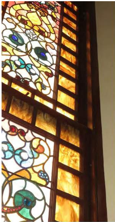
Above: In the border on each side of the figure, two of the sections are double-hung sash which no longer operates.
