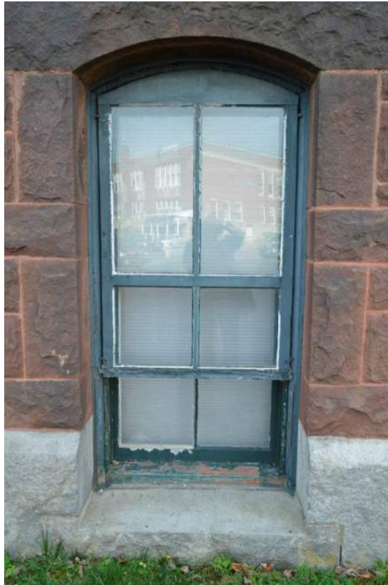
Figure 21 - Wood window sash and surrounding framing and trim should be reglazed and repainted.
