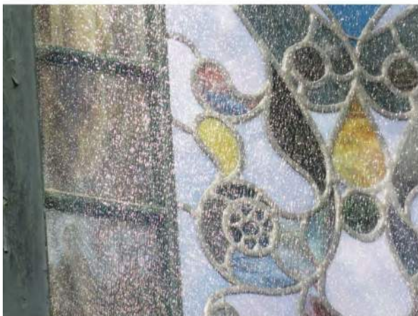
The protective glazing is plastic. It has become very crazed. It should be replaced with laminated glass.
