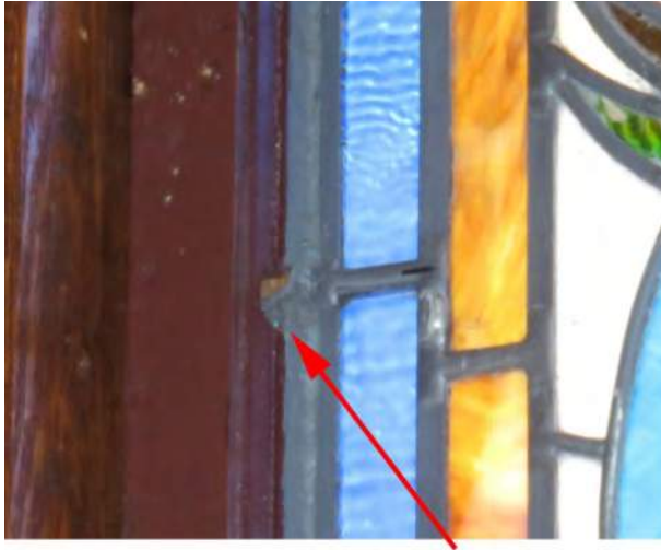
Locations of missing bars are easy to determine because the holes for them still exist in the frame.
