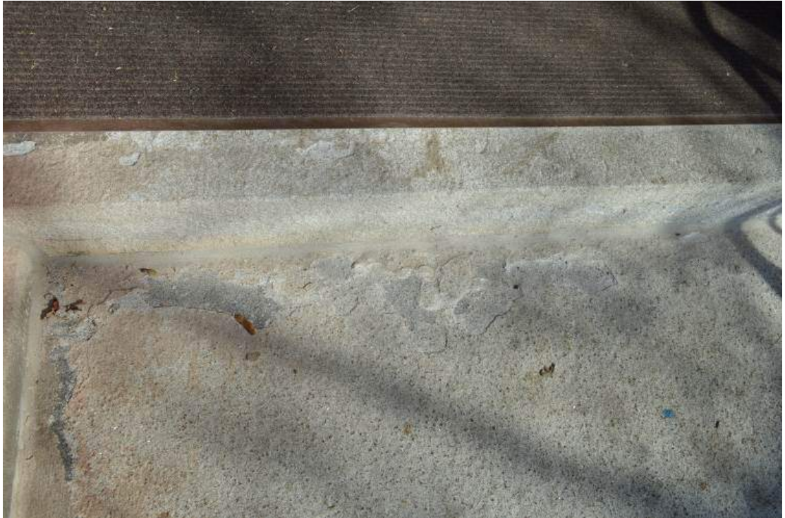
Figure 19 - Sugaring of the granite steps is due to the use of calcium chloride which should be avoided.
